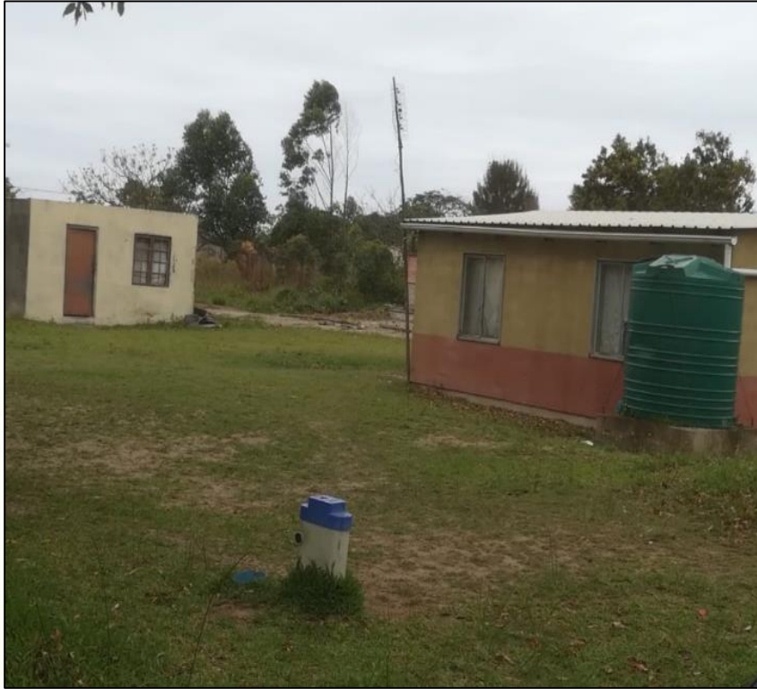
Rain water harvesting – on site
